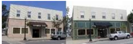
Courtesy photos The photo on the left shows the structure as it looked before remodeling took place. On the right, Fat Tony's displays a fresh paint job, new lights and new signage.
